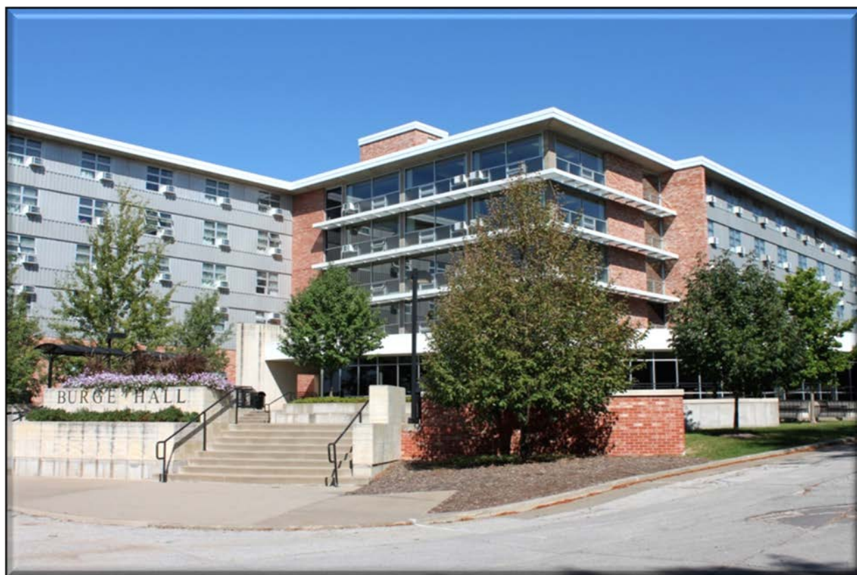
Burge Residence Hall – Update Student Living Spaces (interior only) project built in 1959
