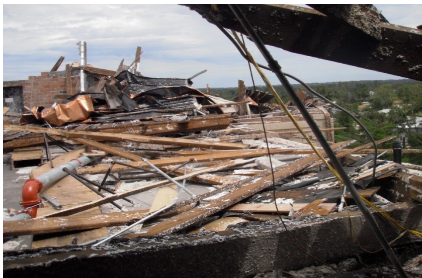
Picture 4– depicts the north wing from on top of the roof
