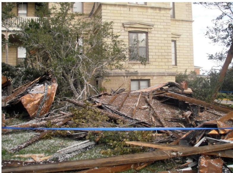
Picture 1 depicts Old Main building debris.
