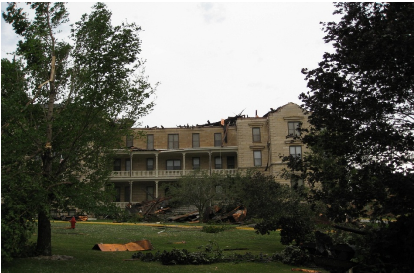
Picture 3 – depicts Old Main north wing roof structure
