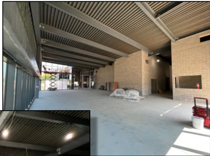
Construction progress, August 2023
