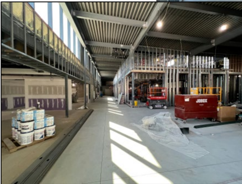
Construction progress, August 2023
