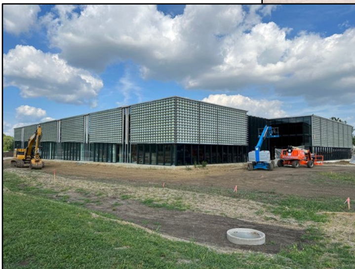
Construction progress: August 2023
