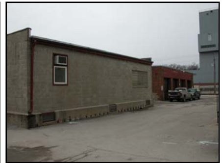
Court St. Building (Util.)
